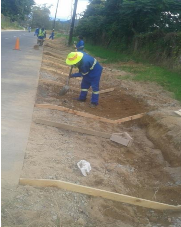
Concrete lined v-drain construction
