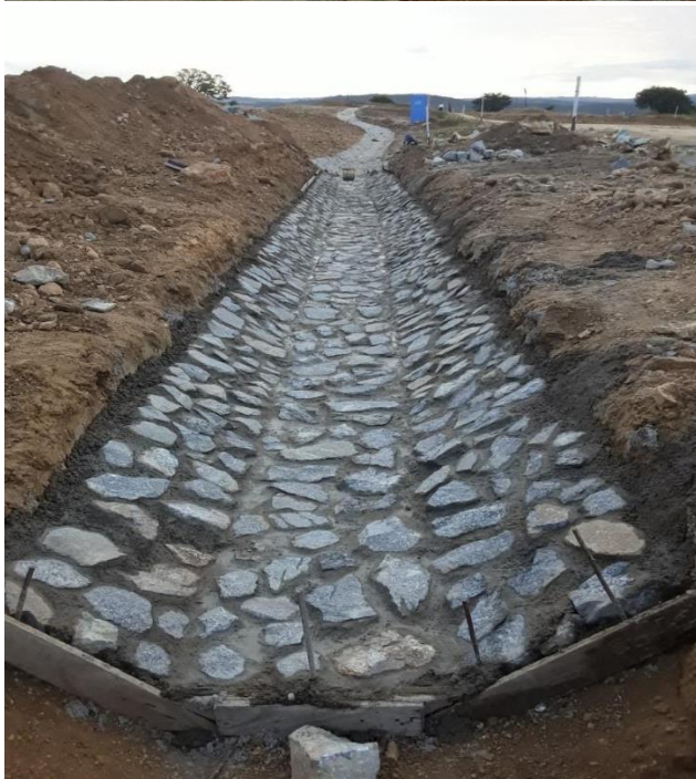
Ngubo Yengwe Construction stone pitching team during construction at Lusip II water project in Big Bend, Eswatini under INES JV, subcontracting under Inyatsi Construction.
